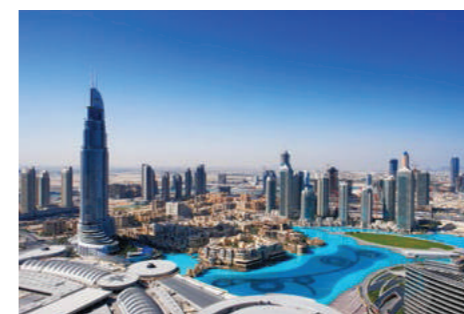
• The constant pressure water supply of the high-rise building and the multi-storey buildings
