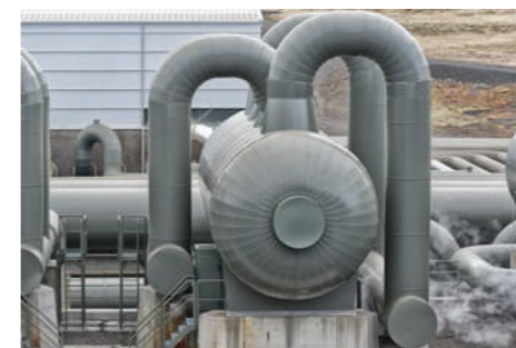
• the water supply pump station
